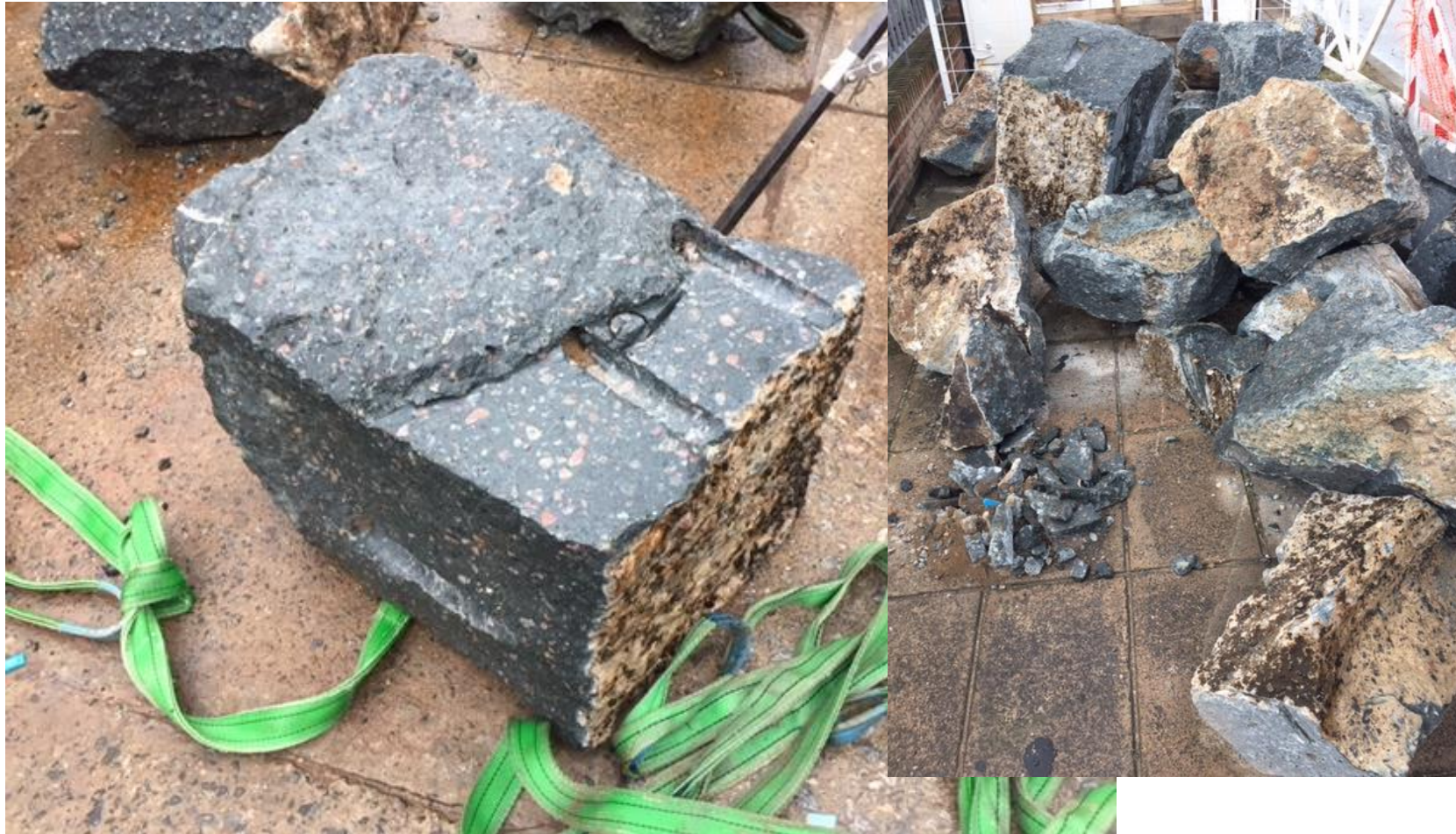
Expansion of concrete sedimentation by diamond saws and hydraulic splitter
